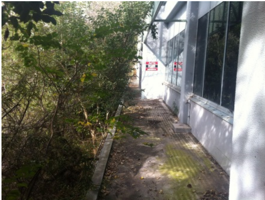
Photo 5.1.8 View of eastern side of building, looking south (rail corridor to the east)
