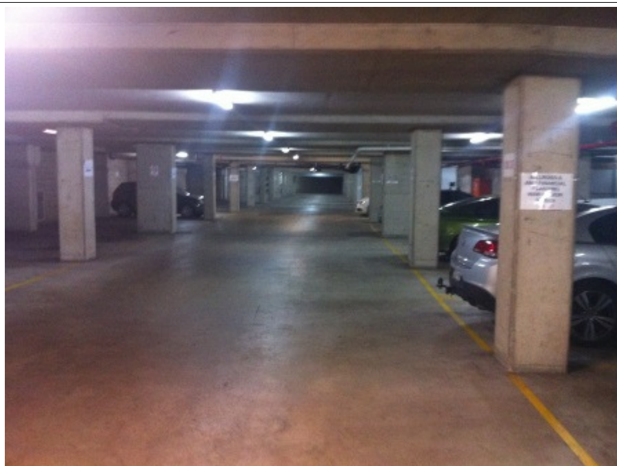
Photo 5.1.6 View of basement level 1 parking
