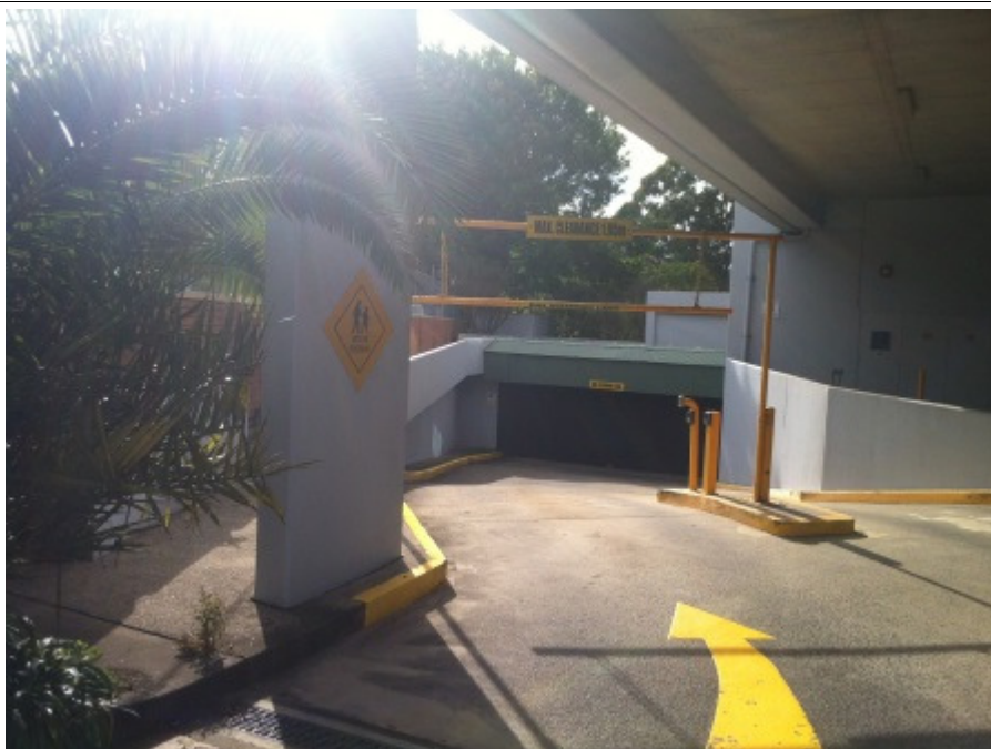
Photo 5.1.5 View of basement carpark entrance driveway at northern end of building
