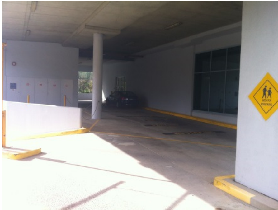
Photo 5.1.4 View of loading dock area
