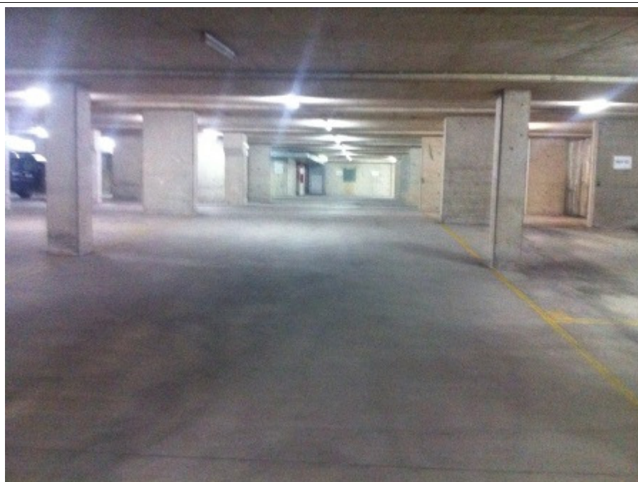
Photo 5.1.7 View of basement level 2 parking
