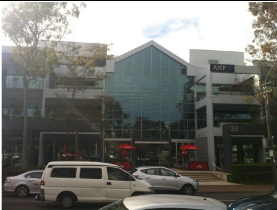
Photo 5.1.1 View of western side of building, looking east
