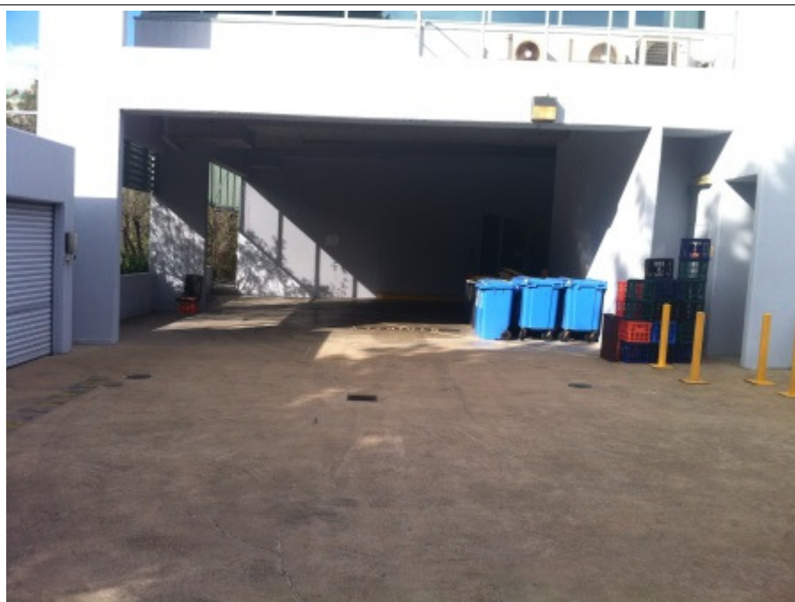
Photo 5.1.3 View of loading dock area
